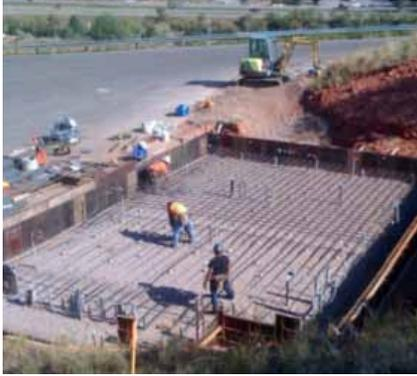
Figure 1. Compressor Station rebar placement
