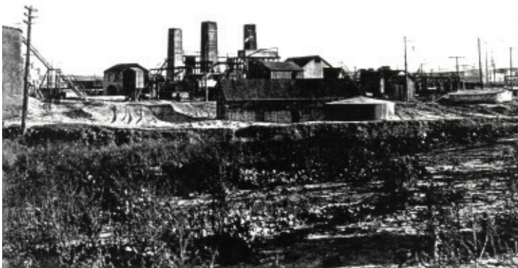
United Refinery, Florence, Colorado
