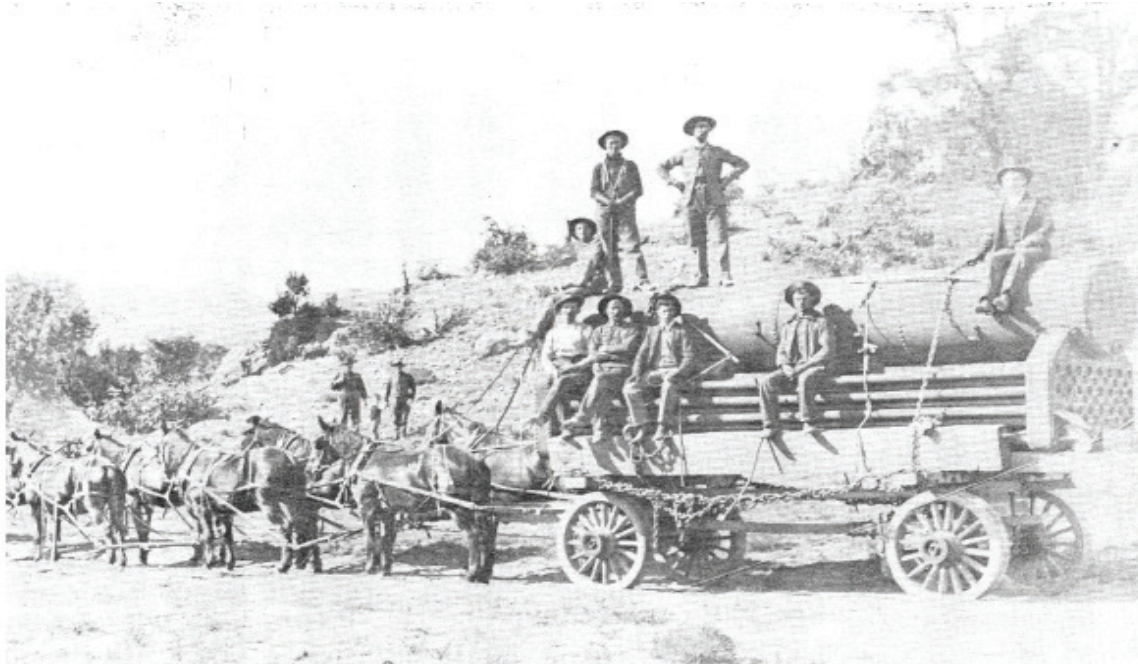
Five teams of horses were used to pull this wagon loaded with a steam boiler used to supply power at the early oil wells, circa 1900
